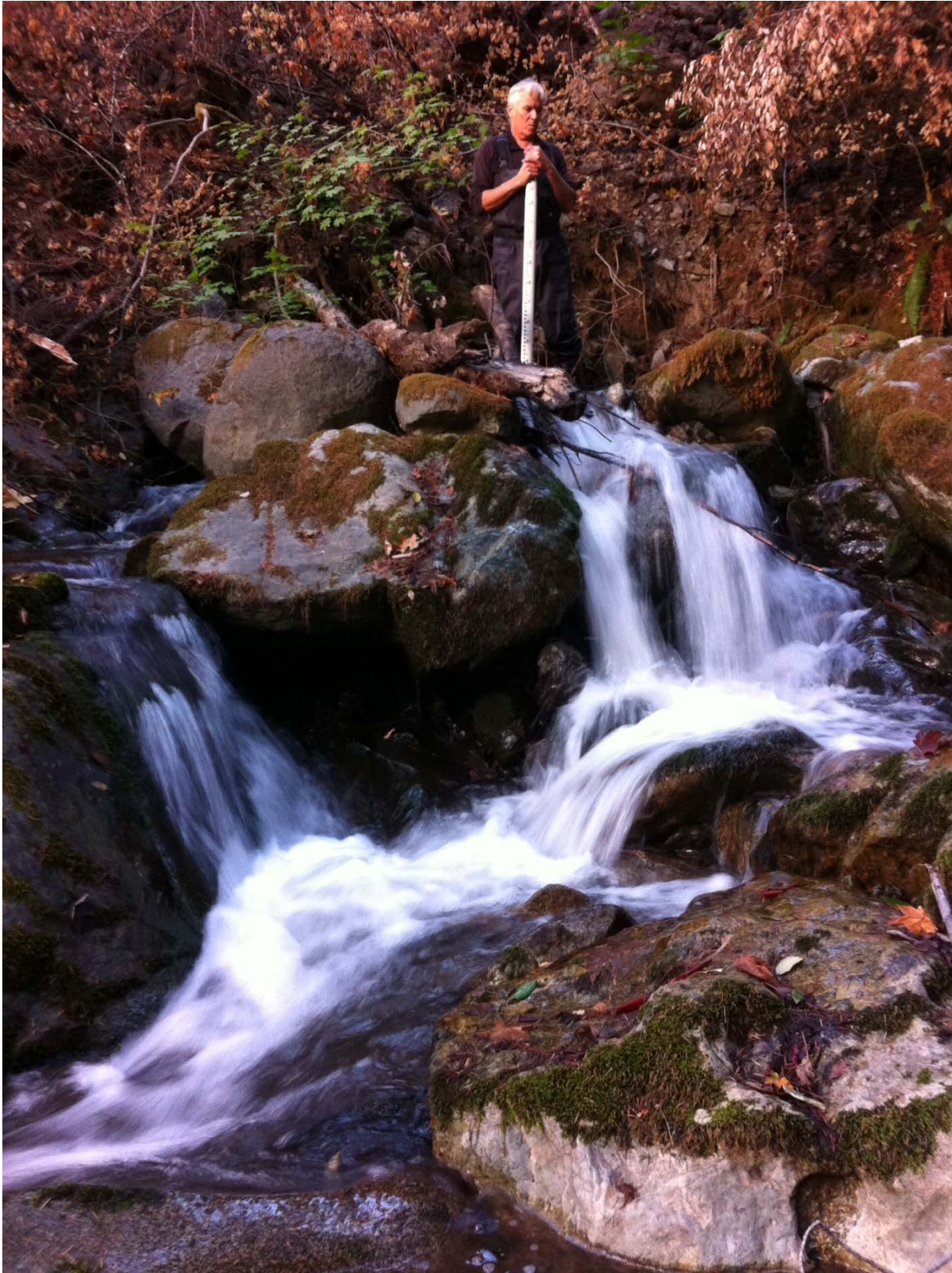
Photo 1. Portion of falls and bedrock chute immediately upstream of the Highway 96 culverts on Stanshaw Creek.
